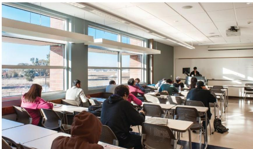
**Figure 2:** The Elk Grove Center in Elk Grove, Calif., is a satellite campus of the Cosumnes River College. The design combines exterior screens and a light shelf to optimize views to outside, solar gain, and natural daylight.
